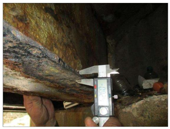
Span 1 Beam 4: (PAR) CORROSION ALONG BOTH FACES OF WEB AND EDGES OF BOTH FLANGES UP TO FULL LENGTH X 8" HIGH DOWN TO 0.216" RESIDUAL WEB, FULL LENGTH X 4" WIDE DOWN TO 0.02" RESIDUAL TOP FLANGE, AND FULL LENGTH X 4" WIDE DOWN TO 0.02" RESIDUAL BOTTOM FLANGE
