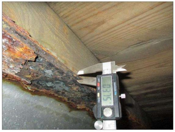
Span 1 Beam 5: (PAR) CORROSION ALONG BOTH FACES OF WEB AND EDGES OF BOTH FLANGES UP TO FULL LENGTH X 2" HIGH DOWN TO 5/16" RESIDUAL WEB, FULL LENGTH X 4" WIDE DOWN TO 0.37" RESIDUAL TOP FLANGE, AND FULL LENGTH X 4" WIDE DOWN 0.08" TO KNIFE'S EDGE RESIDUAL BOTTOM FLANGE Structure: 560149
