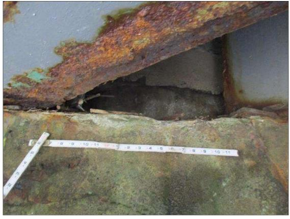
End Bent 1 Abutment: 14" X 2" X 1" DEEP SPALL IN FACE OF CAP BENEATH BAY 5
