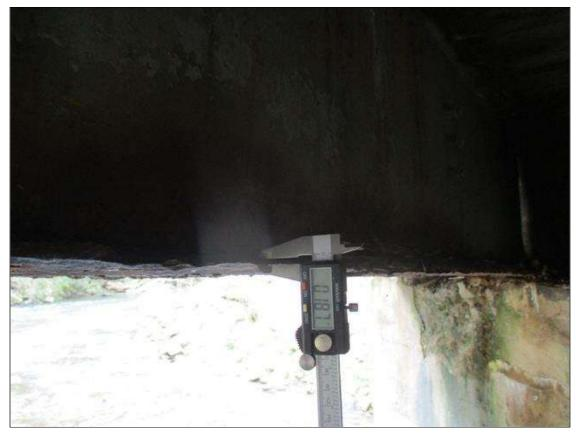
Span 1 Beam 7: (PAR) CORROSION ALONG EDGES OF BOTH FLANGES UP TO FULL LENGTH X 4" WIDE DOWN TO 0.45" RESIDUAL TOP FLANGE, AND UP TO 4' FROM END BENT 1 DOWN TO 0.18" RESIDUAL BOTTOM FLANGE
