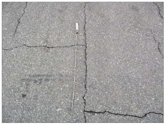
Span 1 Wearing Surface: UP TO 1/4" TRANSVERSE AND LONGITUDINAL CRACKS IN VARIOUS LOCATIONS THROUGHOUT
