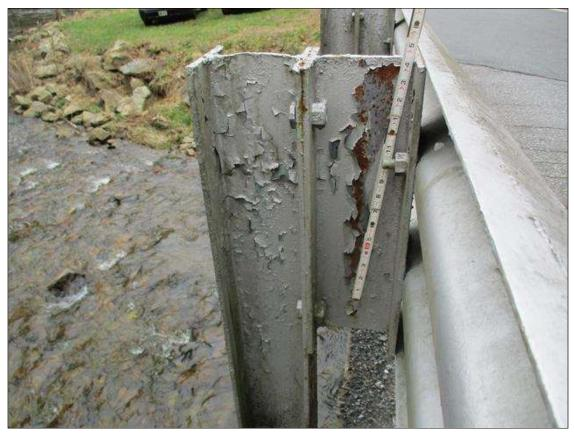
Span 1 Right Bridge Rail: AREAS OF CORROSION IN RAIL POSTS
