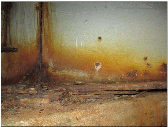
TYPICAL CORROSION WITH SECTION LOSS BEGGINNING ON ALL BEARINGS @ END BENT 1, END BENT 2, & BENT 1
