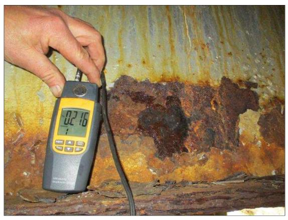
Span 1 Beam 4: (PAR) CORROSION ALONG BOTH FACES OF WEB AND EDGES OF BOTH FLANGES UP TO FULL LENGTH X 8" HIGH DOWN TO 0.216" RESIDUAL WEB, FULL LENGTH X 4" WIDE DOWN TO 0.02" RESIDUAL TOP FLANGE, AND FULL LENGTH X 4" WIDE DOWN TO 0.02" RESIDUAL BOTTOM FLANGE
