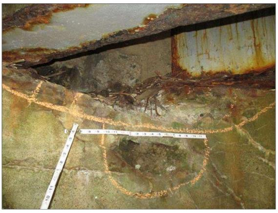
End Bent 1 Abutment: (PAR) 38" X 7" X UP TO 4" DEEP SPALL IN FACE OF CAP BENEATH BEAMS 1 AND 2, WITH 3" X 1" LOSS OF BEARING BELOW BEAM 1
