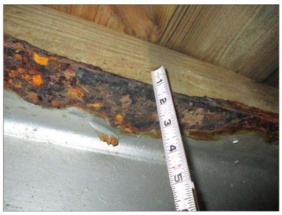
Span 2 Beam 8: (PAR) CORROSION ALONG BOTH FACES OF WEB AND EDGES OF BOTH FLANGES UP TO FULL LENGTH X 4" HIGH DOWN TO 3/8" RESIDUAL WEB, FULL LENGTH X 4" WIDE DOWN TO 0.19" & KNIFE'S EDGE RESIDUAL TOP FLANGE, AND FULL LENGTH X 4" WIDE DOWN TO 0.22" RESIDUAL BOTTOM FLANGE
