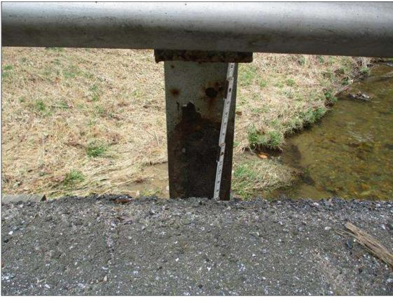
Span 2 Right Bridge Rail - Protective System: AREAS OF DETERIORATED PAINT SYSTEM IN RAIL POSTS
