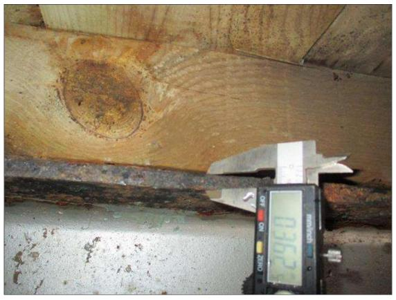
Span 1 Beam 6: (PAR) CORROSION ALONG LEFT FACE OF WEB AND EDGES OF BOTH FLANGES 4' FROM END BENT 1 DOWN TO 0.21" RESIDUAL WEB, 4' FROM END BENT 1 DOWN TO 0.36" RESIDUAL TOP FLANGE, AND NEAR MIDSPAN DOWN TO 0.17" WITH AREAS DOWN TO KNIFE'S EDGE RESIDUAL BOTTOM FLANGE
