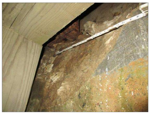
End Bent 2 Abutment: (PAR) FROM BEAM 2 TO BAY 3, 60"x 2"x 6" DEEP SPALL WITH 1" LOSS OF BEAM 3 BEARING. FROM RIGHT END TO BEAM 4, 14' LONG x 21" HIGH FAILED REPAIR WITH UP TO 2" DEEP UNDERMING AT BEAM 5
