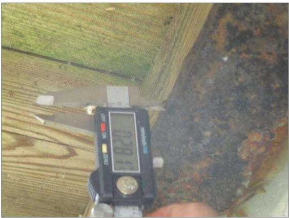
Span 1 Beam 8: (PAR) CORROSION ALONG EDGES OF BOTH FLANGES @ END BENT 1, 0.28" RESIDUAL TOP FLANGE, AND 0.42" RESIDUAL BOTTOM FLANGE
