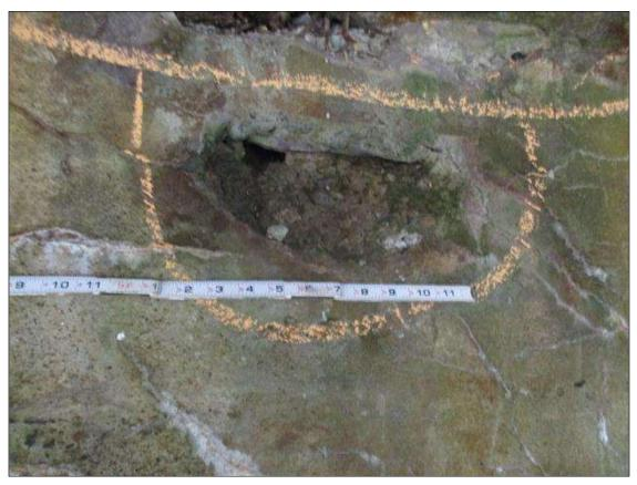
End Bent 1 Abutment: 10" X 5" X 1" DEEP SPALL IN FACE OF BREASTWALL BENEATH BAY 1 NEAR BOTTOM OF CAP
