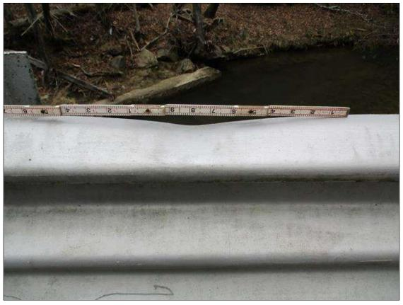
Span 2 Left Bridge Rail: 16" X 1" DEEP DISTORTION IN TOP OF RAIL, APPROXIMATELY 10' FROM PIER
