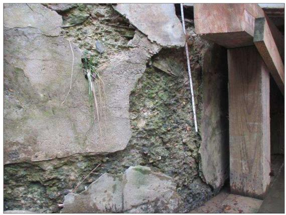
End Bent 2 Abutment: (PAR) BELOW BEAM 1, 16"x 22"x UP TO 10" DEEP SPALL WITH 6" X 5" LOSS OF BEARING IN FACE OF CAP
