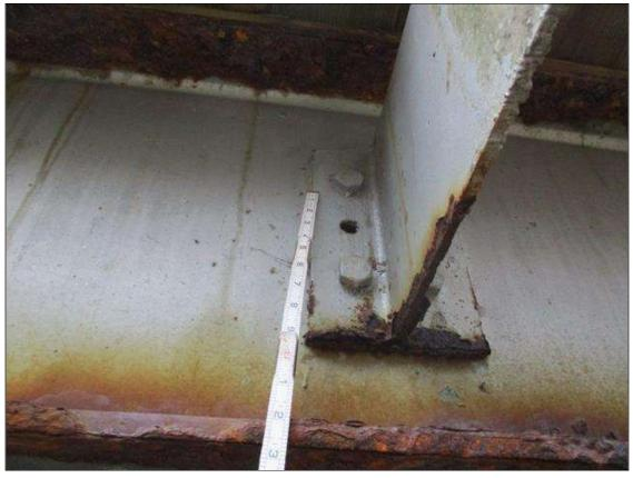
Span 2 Left Bridge Rail: (PAR) RAIL POSTS 5 AND 6, TWO (2) MISSING BOLTS AT CONNECTION TO BEAM 1
