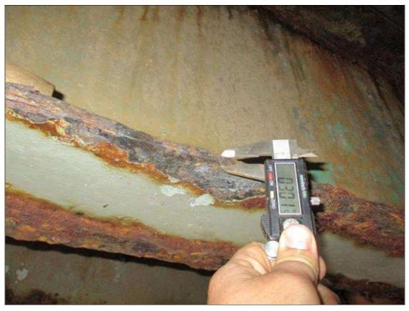
Span 2 Beam 3: (PAR) CORROSION ALONG BOTH FACES OF WEB AND EDGES OF BOTH FLANGES NEAR MIDSPAN DOWN TO 0.25" RESIDUAL WEB, NEAR END BENT 2 0.20" RESIDUAL TOP FLANGE, AND NEAR END BENT 2 DOWN TO 0.30" RESIDUAL BOTTOM FLANGE
