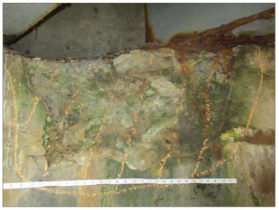
End Bent 1 Abutment: 32" X 16" X UP TO 1" DEEP SPALL IN FACE OF CAP BENEATH BAY 7; NO LOSS OF BEARING NOTED
