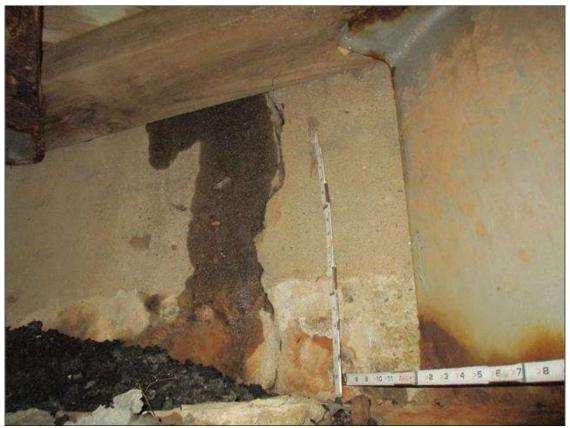
End Bent 2 Abutment: UP TO 24" LONG X 1/4" WIDE VERTICAL CRACKS IN FACE OF BACKWALL IN BAYS 5 AND
