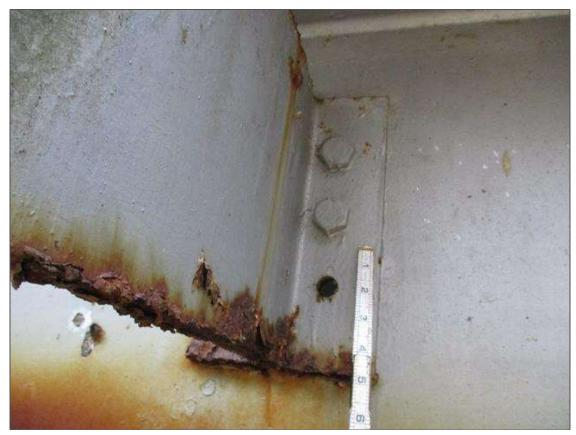
Span 2 Right Bridge Rail: (PAR) MISSING BOLT AT CONNECTION OF RAIL POST TO BEAM 8, APPROXIMATELY 15' FROM ABUTMENT 2
