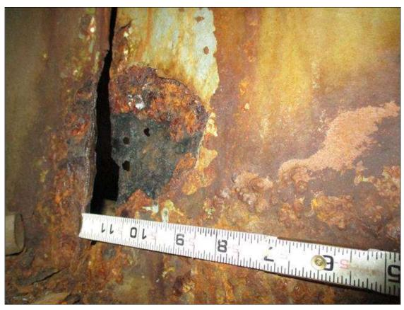
Span 2 Beam 6: (PAR) CORROSION ALONG BOTH FACES OF WEB AND EDGES OF BOTH FLANGES UP TO FULL LENGTH X 4" HIGH AREAS OF KNIFE'S EDGE & 100% SECTION LOSS IN WEB, FULL LENGTH X 4" WIDE DOWN TO 0.25" RESIDUAL TOP FLANGE, AND FULL LENGTH X 4" WIDE DOWN TO 0.17" RESIDUAL BOTTOM FLANGE Structure: 560149
