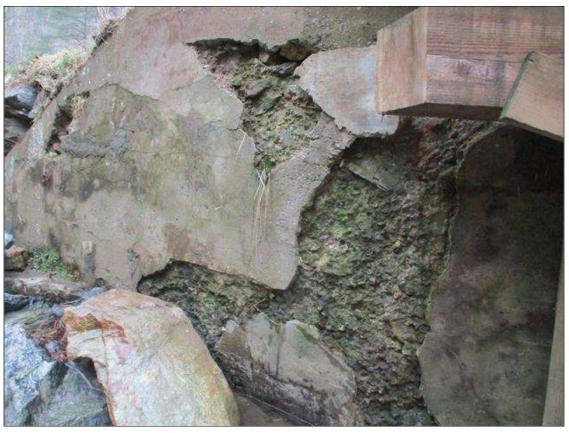
End Bent 2 Abutment: (PAR) NORTHEAST WINGWALL EXTENSION, 11'x 5" AREA OF DELAMINATION FOUR (4) SPALLS UP TO 3'x 3'x 5" DEEP WITH UP TO 1/8" MAP CRACKING WITH EFFLORESCENCE IN FACE
