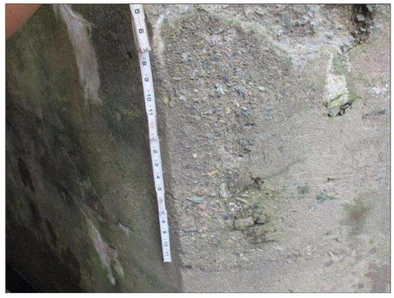
End Bent 1 Abutment: 48' OF UP TO 12" HIGH X 5" DEEP SCALING WITH EXPOSED AGGREGATE THROUGHOUT FACE OF BREASTWALL AT WATER SURFACE WITH UP TO 1/16IN VERTICAL AND HORIZONTAL CRACKS
