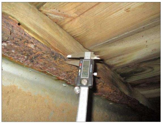
Span 2 Beam 7: (PAR) CORROSION ALONG BOTH FACES OF WEB AND EDGES OF BOTH FLANGES UP TO FULL LENGTH X 4" HIGH DOWN TO 0.24" RESIDUAL WEB, FULL LENGTH X 4" WIDE DOWN TO 0.41" RESIDUAL TOP FLANGE, AND FULL LENGTH X 4" WIDE DOWN TO 0.303" WITH AREAS DOWN TO KNIFE'S EDGE RESIDUAL BOTTOM FLANGE
