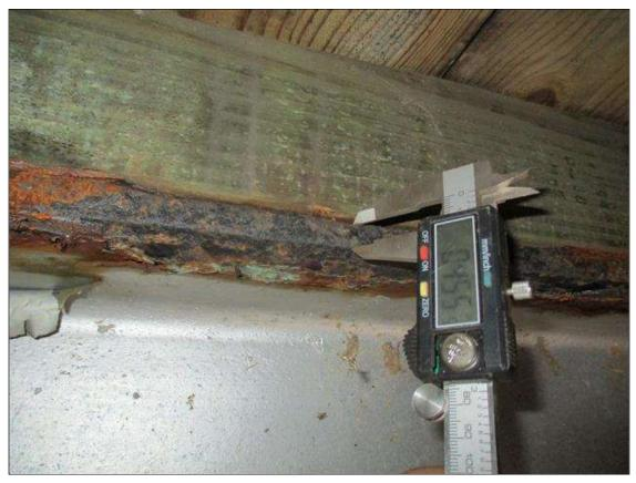
Span 1 Beam 7: (PAR) CORROSION ALONG EDGES OF BOTH FLANGES UP TO FULL LENGTH X 4" WIDE DOWN TO 0.45" RESIDUAL TOP FLANGE, AND UP TO 4' FROM END BENT 1 DOWN TO 0.18" RESIDUAL BOTTOM FLANGE
