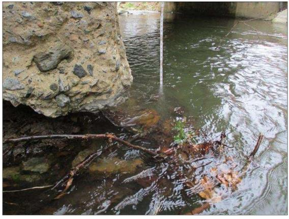
Bent 1 Pier: 25' OF UP TO 36" DEEP SCOUR ALONG BOTH FACES AND UPSTREAM END OF PIER, NO UNDERMINING NOTED
