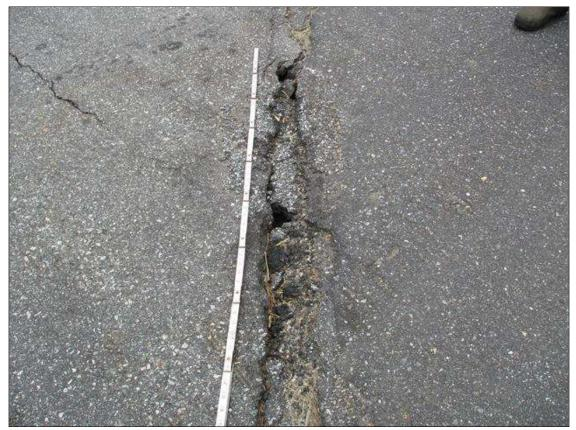
Span 2 Wearing Surface: 12'x 8"x 4" DEEP SPALL & RAVELING OF ASPHALT @ END BENT 2
