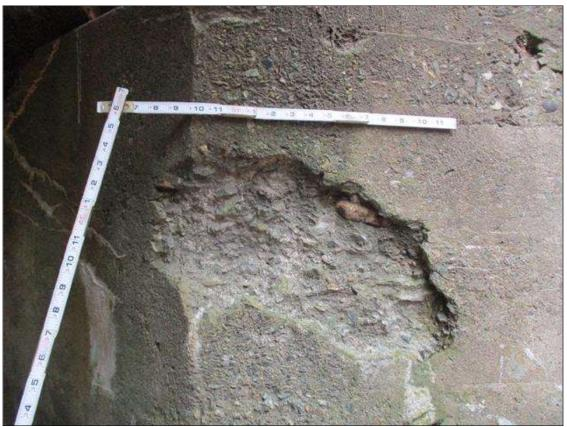
End Bent 1 Abutment: BELOW LEFT OVERHANG NEAR BOTTOM OF BREASTWALL, SPALL 16" X 8" X 1" DEEP
