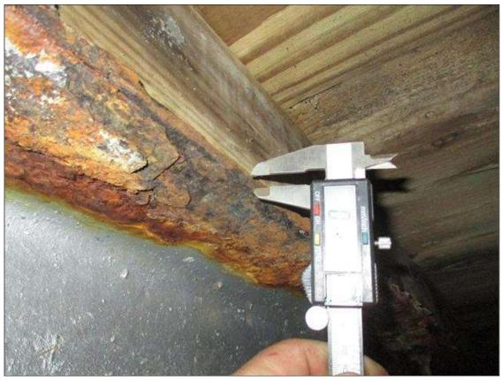
Span 1 Beam 2: (PAR) CORROSION ALONG BOTH FACES OF WEB AND EDGES OF BOTH FLANGES UP TO FULL LENGTH X 4" HIGH DOWN TO 0.25" RESIDUAL WEB, FULL LENGTH X 4" WIDE DOWN TO 0.28" RESIDUAL TOP FLANGE, AND FULL LENGTH X 4" WIDE DOWN TO 0.18" RESIDUAL BOTTOM FLANGE
