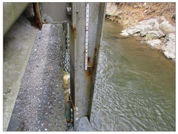
Span 2 Left Bridge Rail - Protective System: AREAS OF DETERIORATED PAINT SYSTEM IN RAIL POSTS
