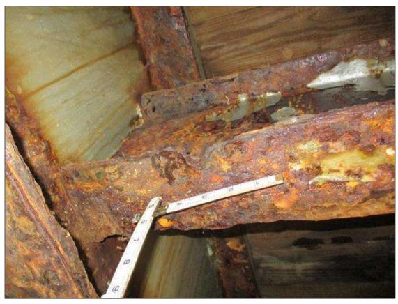
Span 2 Beam 1: (PAR) Bay 1 Diaphragm, 5ft from Pier: CORROSION THROUGHOUT DIAPHRAGM WITH TWO (2) 4" LONG X 2" WIDE HOLES IN TOP FLANGE
