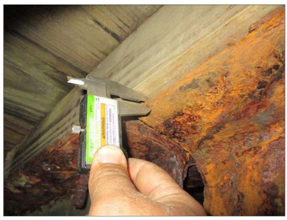
Span 2 Beam 6: (PAR) CORROSION ALONG BOTH FACES OF WEB AND EDGES OF BOTH FLANGES UP TO FULL LENGTH X 4" HIGH AREAS OF KNIFE'S EDGE & 100% SECTION LOSS IN WEB, FULL LENGTH X 4" WIDE DOWN TO 0.25" RESIDUAL TOP FLANGE, AND FULL LENGTH X 4" WIDE DOWN TO 0.17" RESIDUAL BOTTOM FLANGE
