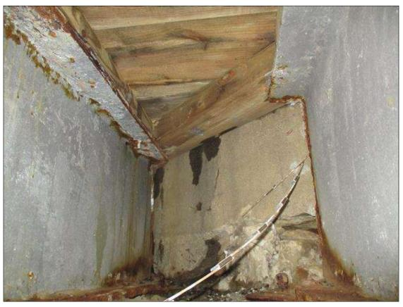
End Bent 2 Abutment: BAY 2 BACKWALL, SPALL 2FT X 10IN X 5IN DEEP
