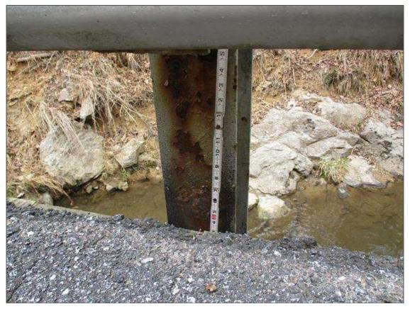
Span 1 Left Bridge Rail: AREAS OF CORROSION IN RAIL POSTS
