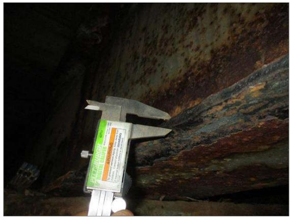
Span 2 Beam 4: (PAR) CORROSION ALONG BOTH FACES OF WEB AND EDGES OF BOTH FLANGES UP TO FULL LENGTH X 16" HIGH DOWN TO 0.24" RESIDUAL WEB, FULL LENGTH X 4" WIDE DOWN TO 0.20" RESIDUAL TOP FLANGE, AND FULL LENGTH X 4" WIDE DOWN TO 0.18" RESIDUAL BOTTOM FLANGE
