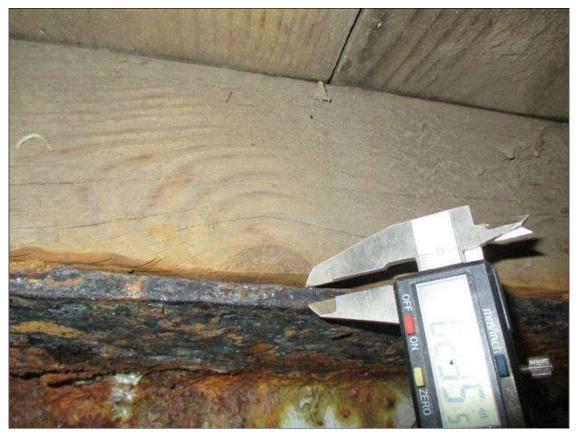
Span 1 Beam 3: (PAR) CORROSION ALONG BOTH FACES OF WEB AND EDGES OF BOTH FLANGES UP TO FULL LENGTH X 10" HIGH DOWN TO 0.16" RESIDUAL WEB, FULL LENGTH X 4" WIDE DOWN TO 0.23" RESIDUAL TOP FLANGE, AND FULL LENGTH X 4" WIDE DOWN TO 0.22" RESIDUAL BOTTOM FLANGE
