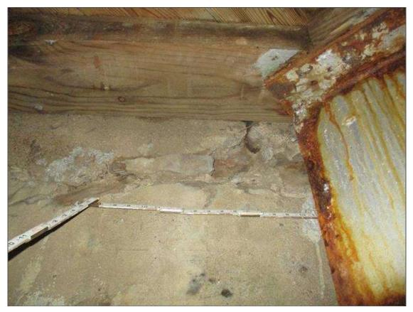
End Bent 1 Abutment: 6" DIAMETER X 2" DEEP SPALL IN FACE OF BACKWALL IN BAY 4
