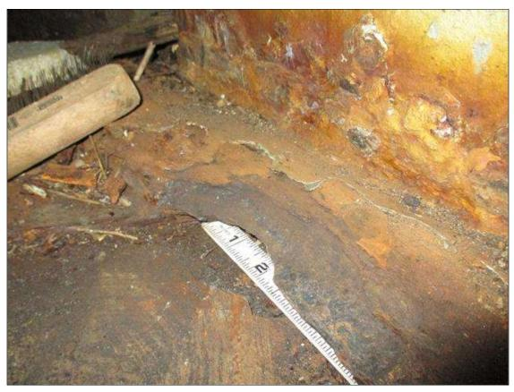
Span 1 Beam 2: (PAR) AT END BENT 1, CORROSION ALONG RIGHT EDGE OF BOTTOM FLANGE WITH 2" LONG X 1/2" WIDE HOLE
