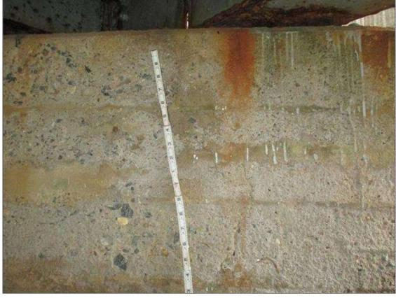
Bent 1 Cap: VERTICAL AND HORIZONTAL HAIRLINE CRACKS IN BOTH FACES OF CAP IN VARIOUS LOCATIONS
