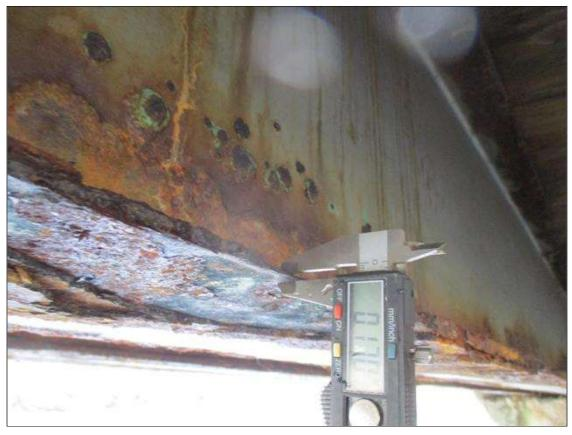
Span 1 Beam 6: (PAR) CORROSION ALONG LEFT FACE OF WEB AND EDGES OF BOTH FLANGES 4' FROM END BENT 1 DOWN TO 0.21" RESIDUAL WEB, 4' FROM END BENT 1 DOWN TO 0.36" RESIDUAL TOP FLANGE, AND NEAR MIDSPAN DOWN TO 0.17" WITH AREAS DOWN TO KNIFE'S EDGE RESIDUAL BOTTOM FLANGE
