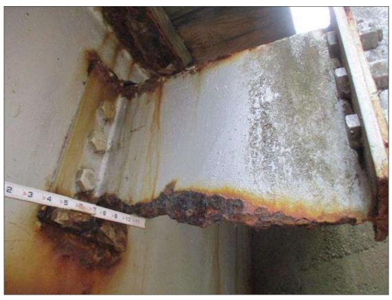
BRIDGE RAIL CONNECTION TO BEAM HAS CORROSION & SECTION LOSS UP TO 100% (TYPICAL ALL BRIDGE RAIL CONNECTIONS)
