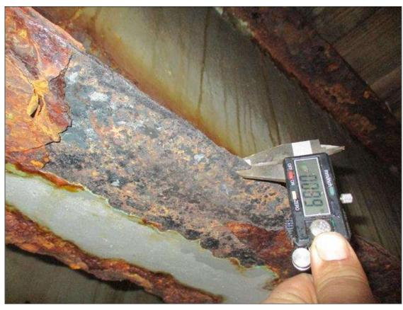
Span 2 Beam 2: (PAR) CORROSION ALONG BOTH FACES OF WEB AND EDGES OF BOTH FLANGES NEAR END BENT 2 DOWN TO 0.24" RESIDUAL WEB, NEAR END BENT 2 DOWN TO 0.23" RESIDUAL TOP FLANGE, AND NEAR END BENT 2 DOWN TO 0.08" RESIDUAL BOTTOM FLANGE
