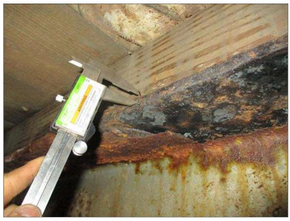
Span 2 Beam 4: (PAR) CORROSION ALONG BOTH FACES OF WEB AND EDGES OF BOTH FLANGES UP TO FULL LENGTH X 16" HIGH DOWN TO 0.24" RESIDUAL WEB, FULL LENGTH X 4" WIDE DOWN TO 0.20" RESIDUAL TOP FLANGE, AND FULL LENGTH X 4" WIDE DOWN TO 0.18" RESIDUAL BOTTOM FLANGE
