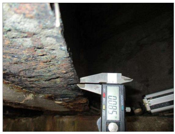
Span 1 Beam 5: (PAR) CORROSION ALONG BOTH FACES OF WEB AND EDGES OF BOTH FLANGES UP TO FULL LENGTH X 2" HIGH DOWN TO 5/16" RESIDUAL WEB, FULL LENGTH X 4" WIDE DOWN TO 0.37" RESIDUAL TOP FLANGE, AND FULL LENGTH X 4" WIDE DOWN 0.08" TO KNIFE'S EDGE RESIDUAL BOTTOM FLANGE
