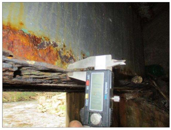
Span 1 Beam 2: (PAR) CORROSION ALONG BOTH FACES OF WEB AND EDGES OF BOTH FLANGES UP TO FULL LENGTH X 4" HIGH DOWN TO 0.25" RESIDUAL WEB, FULL LENGTH X 4" WIDE DOWN TO 0.28" RESIDUAL TOP FLANGE, AND FULL LENGTH X 4" WIDE DOWN TO 0.18" RESIDUAL BOTTOM FLANGE
