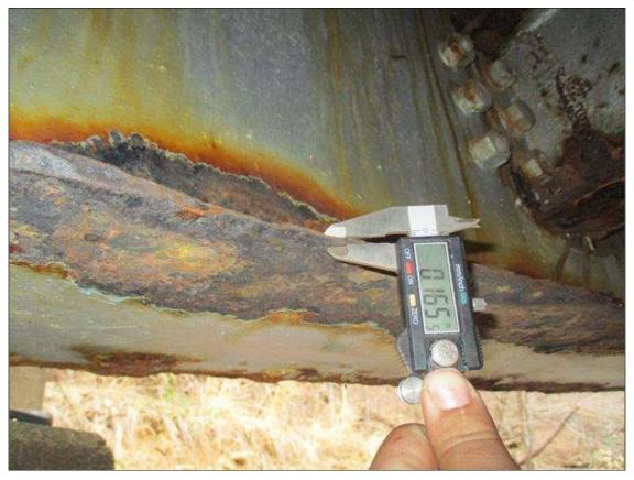
Span 1 Beam 1: (PAR) CORROSION ALONG BOTH FACES OF WEB AND EDGES OF BOTH FLANGES UP TO FULL LENGTH X 4" HIGH DOWN TO 1/4" RESIDUAL WEB, FULL LENGTH X 4" WIDE DOWN TO KNIFE'S EDGE RESIDUAL TOP FLANGE, AND FULL LENGTH X 4" WIDE DOWN TO KNIFE'S EDGE 0.16" BOTTOM FLANGE
