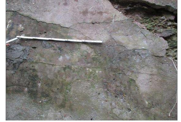
End Bent 2 Abutment: 36" LONG X 60" HIGH X UP TO 8" DEEP SPALL IN FACE OF BREASTWALL AT RIGHT END
