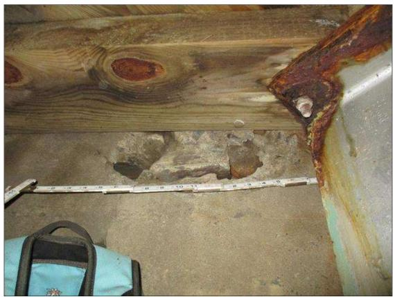
End Bent 1 Abutment: 9" X 5" X 2" DEEP SPALL IN FACE OF BACKWALL IN BAY 6
