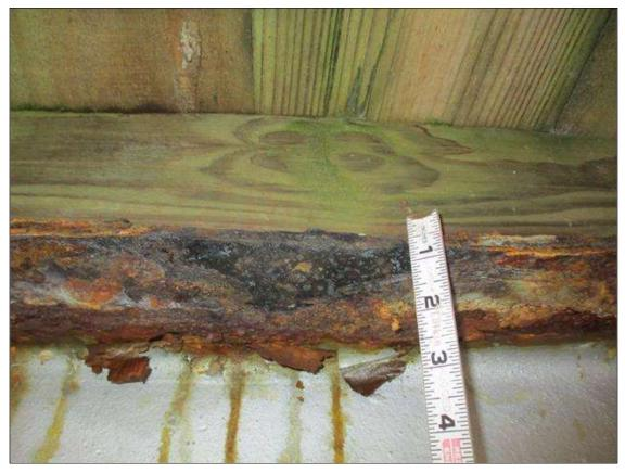
Span 1 Beam 1: (PAR) CORROSION ALONG BOTH FACES OF WEB AND EDGES OF BOTH FLANGES UP TO FULL LENGTH X 4" HIGH DOWN TO 1/4" RESIDUAL WEB, FULL LENGTH X 4" WIDE DOWN TO KNIFE'S EDGE RESIDUAL TOP FLANGE, AND FULL LENGTH X 4" WIDE DOWN TO KNIFE'S EDGE 0.16" BOTTOM FLANGE County: MADISON
