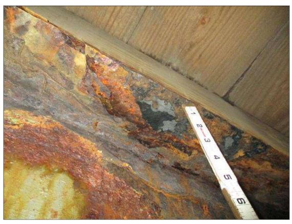
Span 2 Beam 5: (PAR) CORROSION ALONG BOTH FACES OF WEB AND EDGES OF BOTH FLANGES 8' FROM BENT 1 AND @ BEAM END PATCH HAS 100% SECTION LOSS IN WEB, FULL LENGTH X 4" WIDE DOWN TO 0.20" & KNIFE'S EDGE RESIDUAL TOP FLANGE, AND FULL LENGTH X 4" WIDE AREAS DOWN TO KNIFE'S EDGE & 100% SECTION LOSS IN BOTTOM FLANGE
