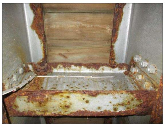
Span 2 Beam 7: (PAR) Span 2 Bay 7 Diaphragm 10ft from Pier: CORROSION THROUGHOUT DIAPHRAGM WITH TWO (2) 3" LONG X 1" WIDE HOLES IN TOP FLANGE, TWO (2) 3" LONG X 1" WIDE HOLES IN BOTTOM FLANGE, AND 3" HIGH X 1 1/2" WIDE HOLE IN WEB
