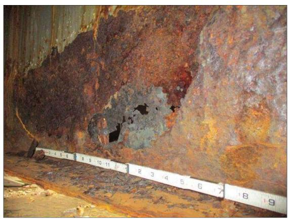
Span 2 Beam 5: (PAR) CORROSION ALONG BOTH FACES OF WEB AND EDGES OF BOTH FLANGES 8' FROM BENT 1 AND @ BEAM END PATCH HAS 100% SECTION LOSS IN WEB, FULL LENGTH X 4" WIDE DOWN TO 0.20" & KNIFE'S EDGE RESIDUAL TOP FLANGE, AND FULL LENGTH X 4" WIDE AREAS DOWN TO KNIFE'S EDGE & 100% SECTION LOSS IN BOTTOM FLANGE Structure: 560149
