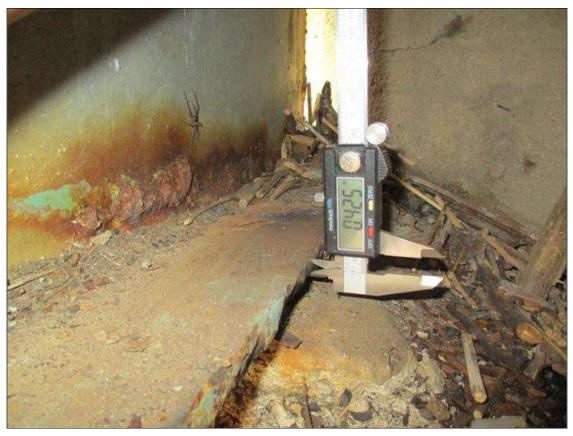
Span 1 Beam 8: (PAR) CORROSION ALONG EDGES OF BOTH FLANGES @ END BENT 1, 0.28" RESIDUAL TOP FLANGE, AND 0.42" RESIDUAL BOTTOM FLANGE
