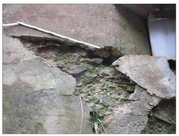
End Bent 2 Abutment: TOP MIDDLE OF LEFT BREAST WALL, 3'x 2'x 4" DEEP SPALL
