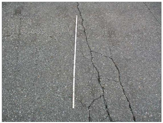
Span 2 Wearing Surface: UP TO 1/4" TRANSVERSE AND LONGITUDINAL CRACKS IN VARIOUS LOCATIONS THROUGHOUT, CRACKS NEAR ABUTMENT 2 FILL FACE
