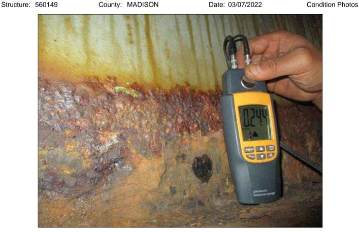
Span 2 Beam 2: (PAR) CORROSION ALONG BOTH FACES OF WEB AND EDGES OF BOTH FLANGES NEAR END BENT 2 DOWN TO 0.24" RESIDUAL WEB, NEAR END BENT 2 DOWN TO 0.23" RESIDUAL TOP FLANGE, AND NEAR END BENT 2 DOWN TO 0.08" RESIDUAL BOTTOM FLANGE
