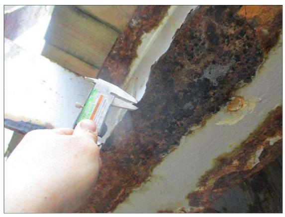
Span 2 Beam 1: (PAR) CORROSION ALOG BOTH FACES OF WEB AND EDGES OF BOTH FLANGES UP TO FULL LENGTH X 4" HIGH DOWN TO 1/4" RESIDUAL WEB, NEAR MIDSPAN DOWN TO 0.23 RESIDUAL IN TOP FLANGE AND DOWN TO 0.18" RESIDUAL IN BOTTOM FLANGE, 5' FROM END BENT 2 HAS 100% SECTION LOSS FOR 1' IN BOTTOM LEFT FLANGE
